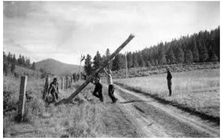
Workers under the old CCC
